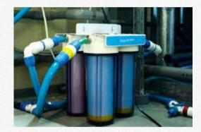
Two NA WATER, installed in the back of the 7m wide tank, were interlinked for corresponding with high amount of water-change; one is loaded with a sediment pre-filter, and a carbon filter, and the other with two Cation Filters.
